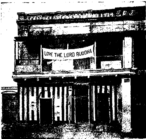
Society Headquarters at 4A, Bankim Chatterjee St. Demolished for erection of the Vihara
